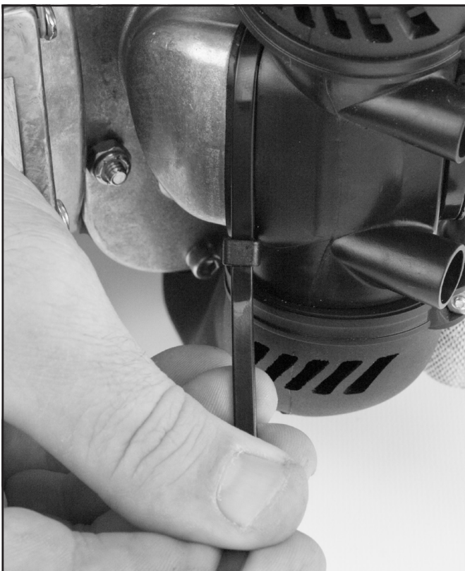
Carefully tighten tie wrap.
