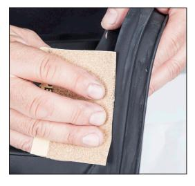
1. Using 120 grit sandpaper, sand a 1 ¼ inch (3.175 cm) wide strip all the way around the outside edge of the face seal. This 1 ¼ inch (3.175 cm) strip will be the mating surface for the neoprene hood
